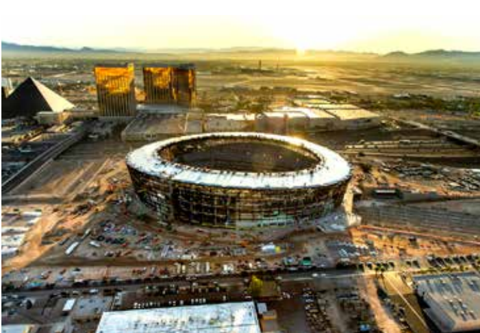
The new Raiders Stadium, a.k.a. "The Trex Dome"
